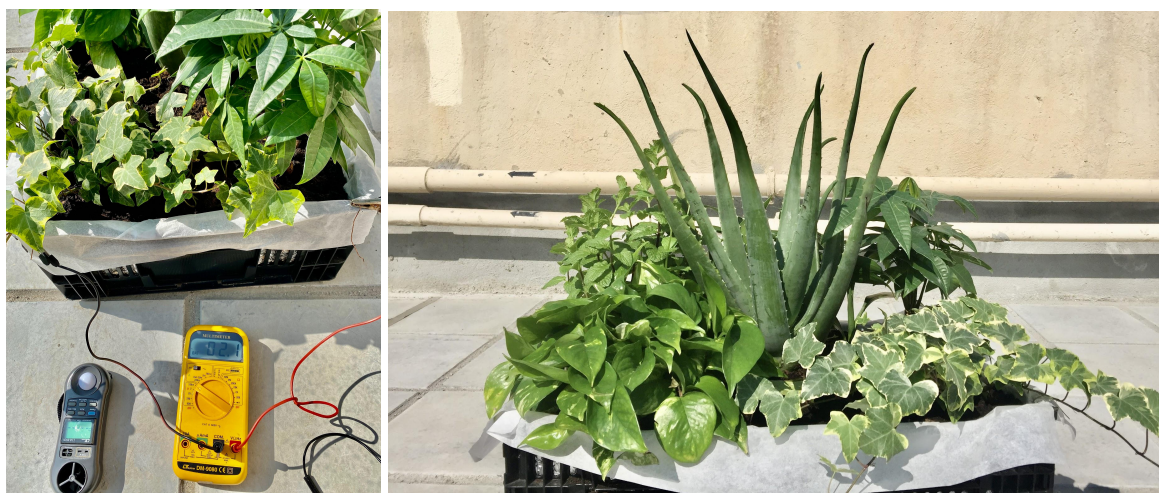
Fig. 2.16 The device diagram of Power Plant in Plant with plants in a relatively larger area
